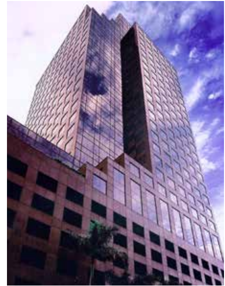
110 Tower - Photo Courtesy of Transwestern
